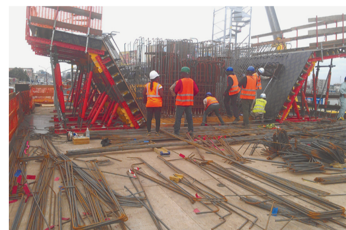
Construction of the Japan-Côte d'Ivoire Friendship Interchange in Abidjan is underway. JAPAN INTERNATIONAL COOPERATION AGENCY
